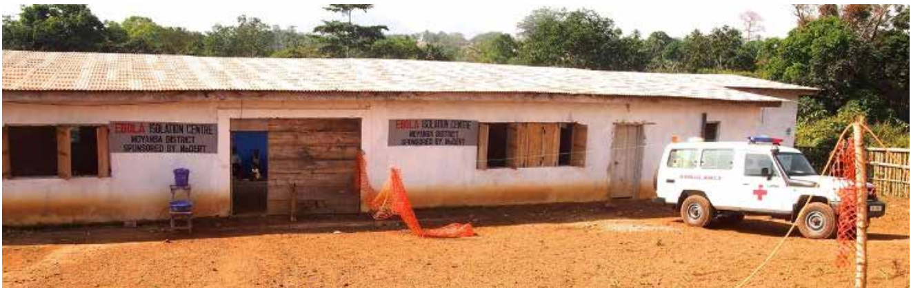
The old Ebola Hospital at Moyamba
