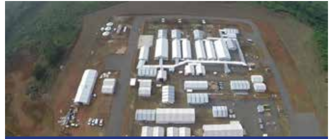
Aerial view of the new 100 bed Ebola hospital
