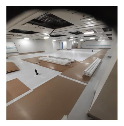
Floor protection being installed after resin has been laid.
