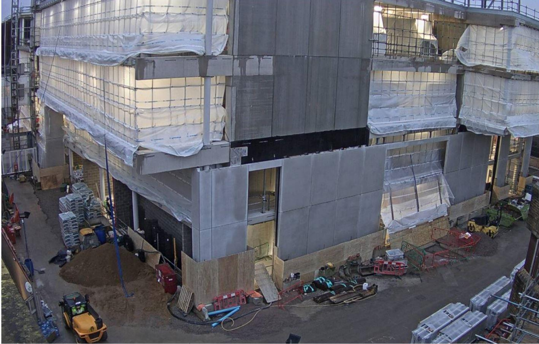
Biochemistry Phase 2 construction - looking north-west 2019-12-10 16:04:42
