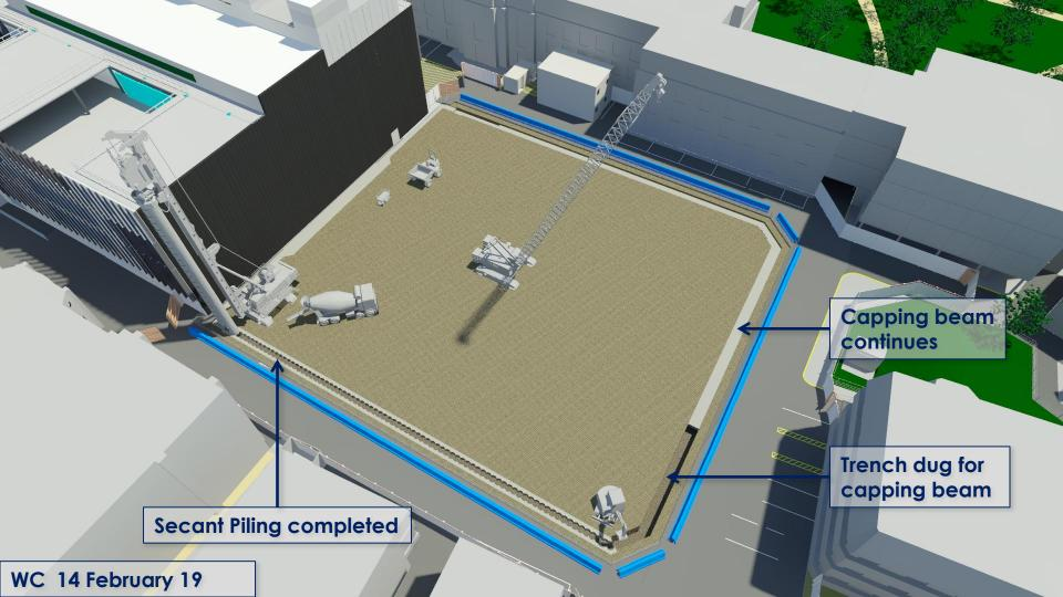
Excavation to underside of capping beam – approx 1.5m depth (+61.05m)
