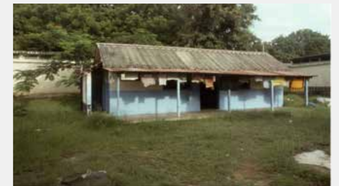
Figure 3a: How to build a paediatric ITU in three months in Kilifi Kenya, 1990 (before)
