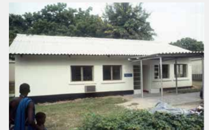
Figure 4b: How to build a paediatric ITU in three months in Kilifi Kenya, 1990 (after)
